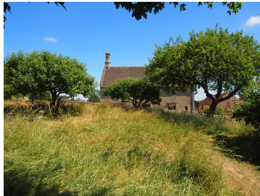
Photo 4: The immediate setting to the west comprises the current orchard, which includes the celebrated 'Newton's Apple Tree' surrounded by a low wicker fence. The orchard contains several mature apple trees, as well as paths and a bench. In some views the farmyard is visible beyond the house, and there are also glimpses of the roofs of properties along Woolsthorpe Road, seen across Stoke Rochford Field/ Beeson's Close.
