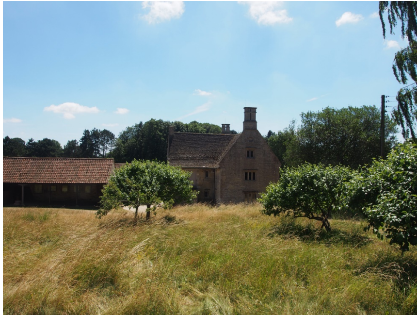
Photo 1: The immediate setting of the property to the north comprises a fairly open walled area. It was formerly an orchard or kitchen garden, and has recently been replanted with apple trees. With the exception of the overhead wires and pole, this is a rural view without modern features. A copse can be seen behind the house and forms the horizon.
