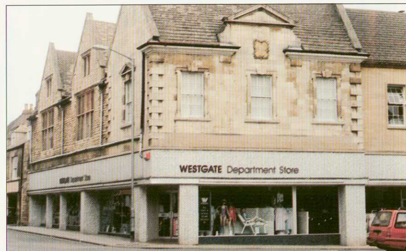
4.1 Poor shopfronts do not reflect the scale and proportion of the building.
