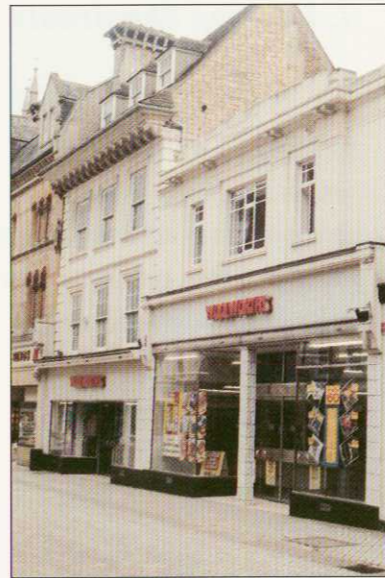
4.1 Uniform designs disregard the individual character of the building.
