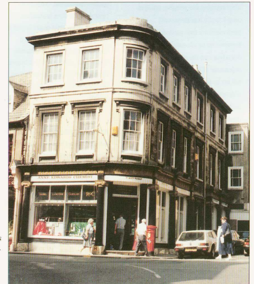
10.2 Conspicuous alarm boxes can spoil a good facade.
