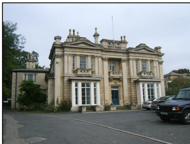
Fig. 16. Rock House and adjacent petrol station.
