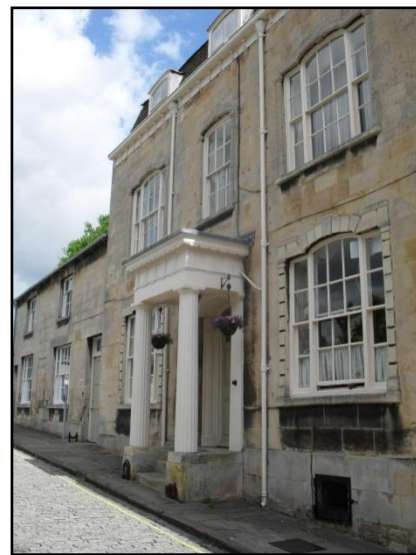
Fig. 15. Classical façade, No. 9 Barn Hill.
