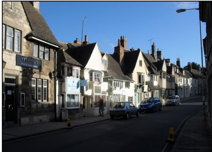
Fig. 3. Medieval buildings on the north side of St Paul's Street
