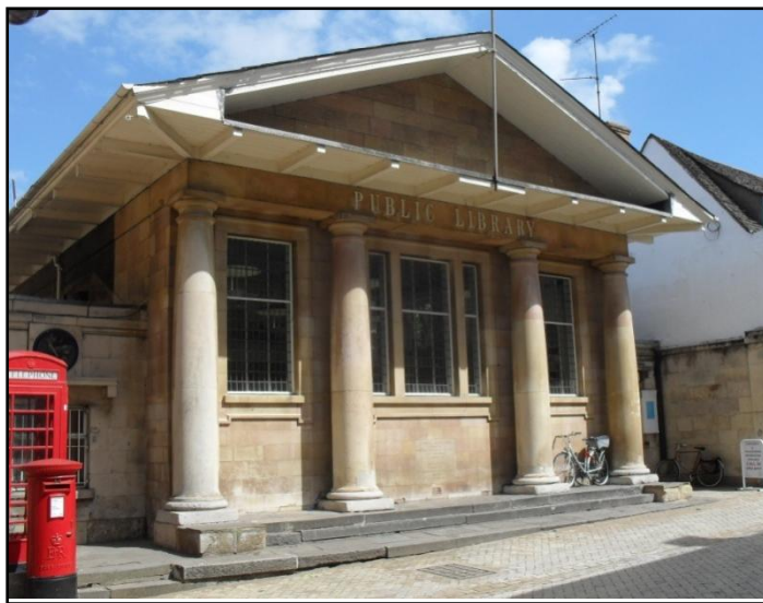
Fig. 6. The portico entrance to the shambles on High Street, converted to a library in 1906.
