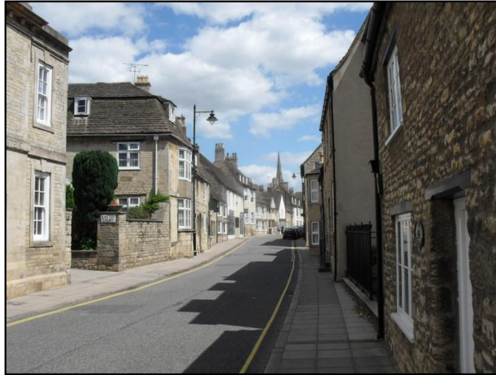
Fig. 17. Eastern view along St Peters Street.
