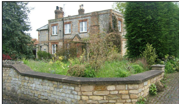
Fig.8 Rectory Cottage, Church Lane is a 19 th century detached residence, constructed of buff brick with contrasting red brick detailing is a 'positive unlisted' building in the conservation area.
