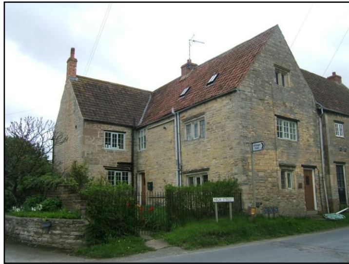
Fig.5 Nos. 39 & 41 High Street (Grade II), an imposing 3 storey building with attractive window details such as stone mullions.
