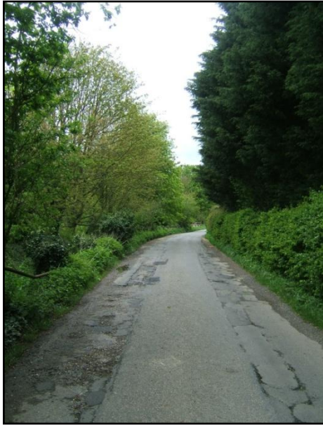
Fig.6 View westwards along Fishpool dike is constrained by hedgerows contributing to linear views.
