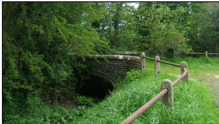
Fig. 10 The concrete and metal fence at Fishpool Dike would benefit from replacement with a traditional wooden post and rail fence.
