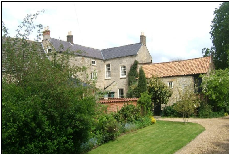
Fig.3 Coverley House (Grade II), on the south east of Church Street; the large three storey detached house is located within a good sized plot that extends to Fishpool Dike makes a strong contribution to Church Lane and the conservation area as a whole.
