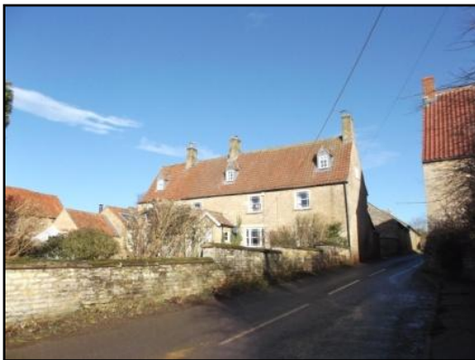
Fig.12 Far Farm, constructed of coursed rubble stone, pantile roof, dormer windows and an attractive boundary
