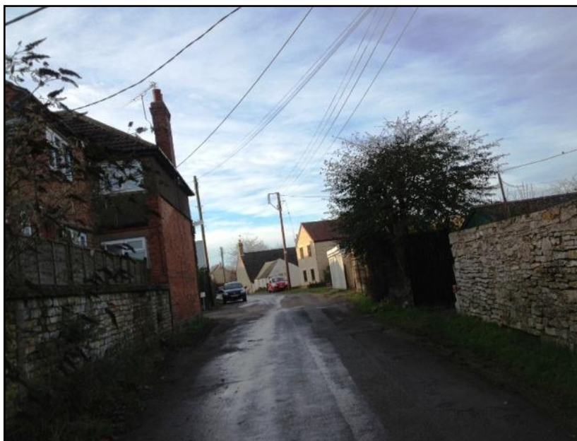
Fig.14 Plethora of overhead cables at Lords Lane detracting from the character and appearance of the conservation area.
