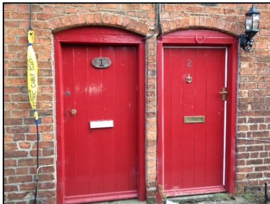
Fig.3 Timber panel doors at Blue Town
