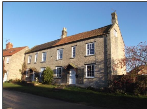
Fig.5 'Stone House' and 'Green View', Church Street which are typical of Skillington, with coursed limestone walling, pantile roof and traditional timber sash windows (Grade II).
