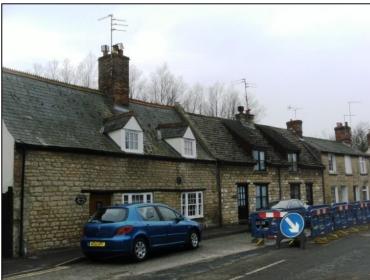
Fig 2. Small scale cottages on the south side of Stamford road, Collywestern tiles are a common roofing material
