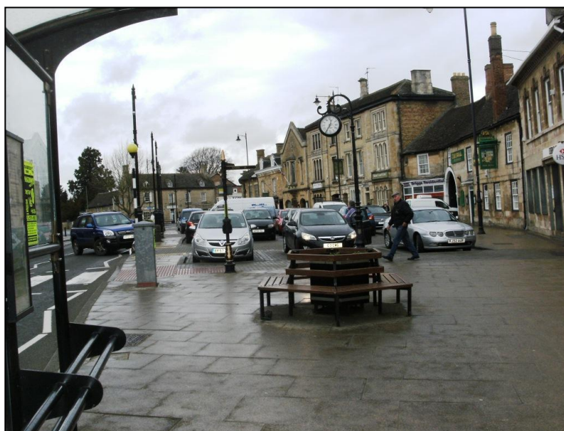
Fig. 16 The attractive buildings within the town centre are undermined by the profusion of street furniture.
