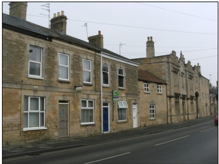
Fig. 18 The replacement of traditional wooden windows, with UPVC, causes cumulative harm to the character of the conservation area, and is particularly noticeable on groups of buildings such as terraces.
