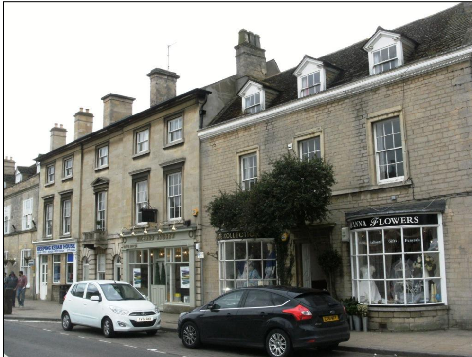
Fig.5 High Street (south side) comprises of large three storey buildings, using classical detailing
