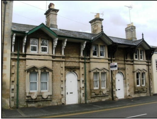
Fig. 7 Nos. 37 & 39 High Street with decorative gables supported by Timber Brackets, prominent chimneys and doorways are an attractive grouping.
