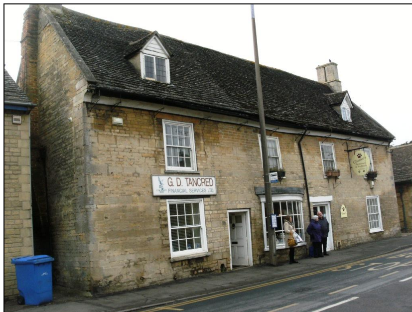
Fig 6. 102 & 104 Church Street (Grade II) are typical of the architecture found within Market Deeping, constructed of rubble stone, Collywestern roof with dormer, prominent chimneys and a bowed window.
