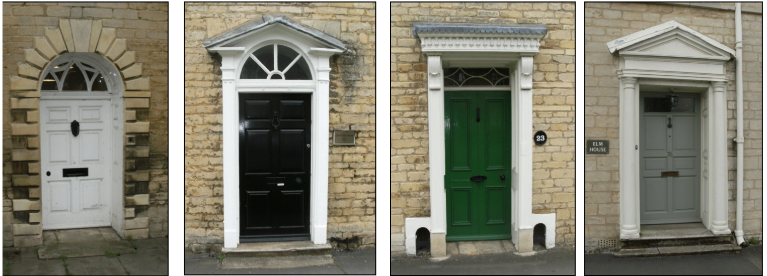
Fig. 9 From left to right: No. 35 Church Street (Holland House) with a 6 panel door, fanlight above and set within a rusticated quoin surround, 21 Church Street (Courtfield House) with fanlight and pediment above and 6 panel door, very typical of Georgian design, No.23 Church Street with a rectangular light and decorative hood above and 76 Church Street (Elm House). All of the doors are associated with town houses on Church Street that are Grade II listed, constructed during period of growing wealth for the market town following the construction of the Stamford Canal.
