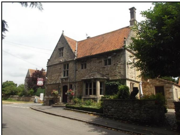
Fig.6 Brownlow Arms (Grade II) in a Tudoresque style built in 1852 and part of the former Brownlow estate.
