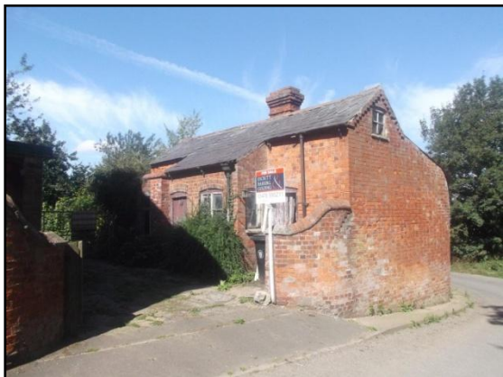
Fig.16 Outbuildings at the cottage, display an exuberant style with decorative chimney stacks, typical of the design found within the 'Brownlow' estate
