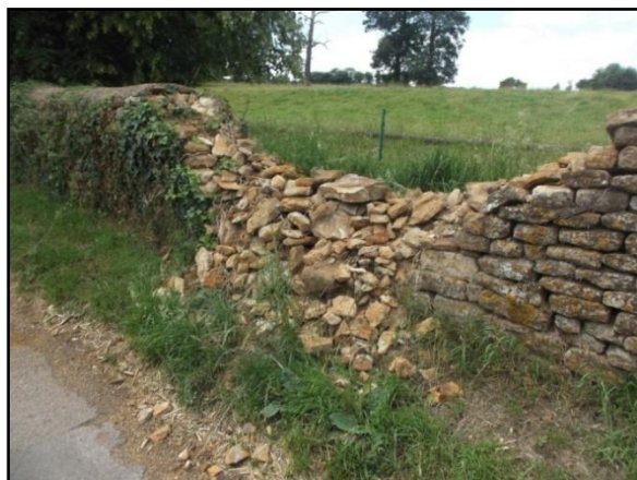
Fig.17 Boundary walls make a positive contribution to the conservation area and it is unfortunate that there are a number of examples in need of repair. Growing ivy appears to be worsening the problem.
