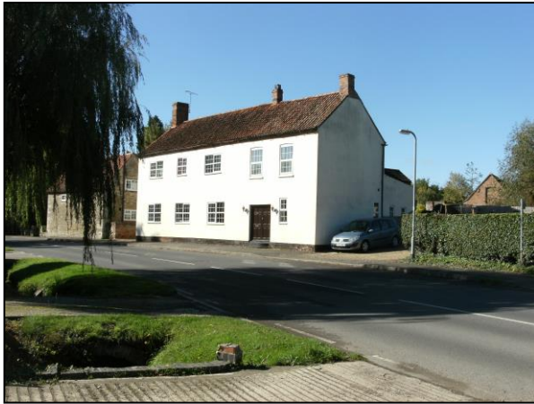
Fig.15 21 & 25 High Street. Loss of character with modern inappropriate windows and doors and render over masonry.
