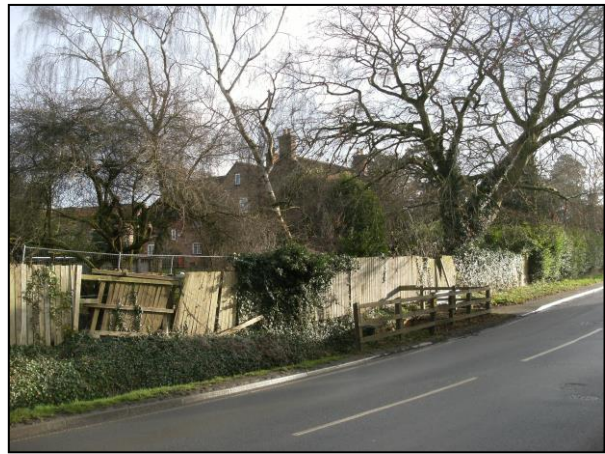
Fig.8 Dilapidated fencing to Abbots Farm frontage
