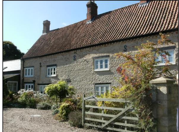
Fig.14 Early eighteenth century Church Cottage, No.1 Church Lane.
