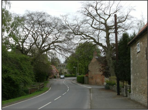
Fig.2 High Street. View south to Church of St. Andrew.
