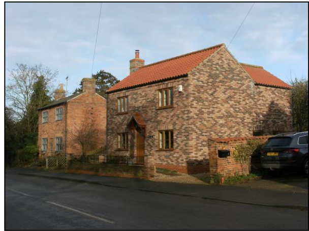
Fig.16 No.6 High Street. Sympathetically designed infill off High Street.
