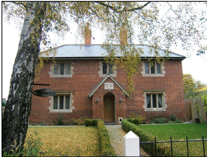
Fig. 2 Netherlea (Grade II), No. 20 High Street demonstrates later design qualities having been built by John Sherwin Gregory. The building bears a plaque with his initials.
