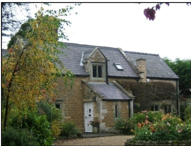
Fig.12 No.2 West End, constructed in the Harlaxton estate style of coursed ironstone with Ashlar dressings.
