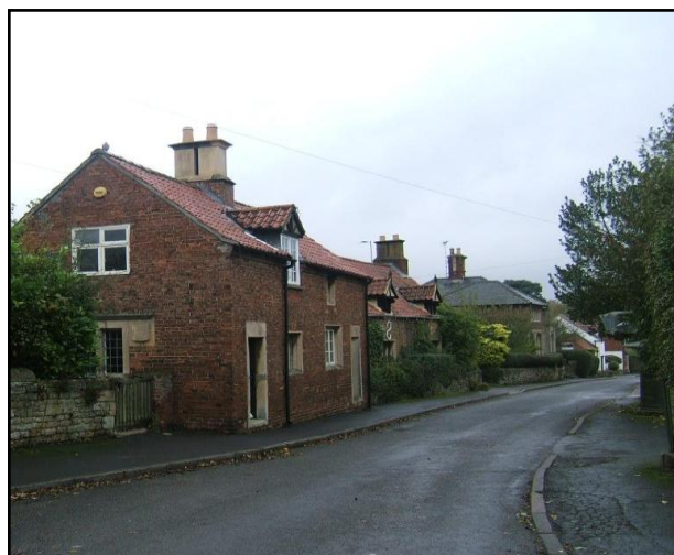
Fig.4 Church Street displays a more traditional plan form with narrow footways and buildings aligned close to footways.
