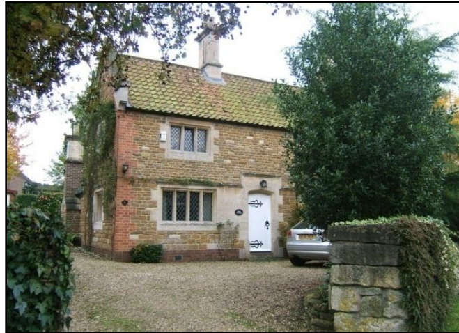
Fig.9 Stone is a common material used for decoration, particularly for door surrounds, mullions, chimneys as at The Tudor House, No.1 Pond Street
