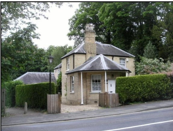
South Lodge, Stonebridge House.
