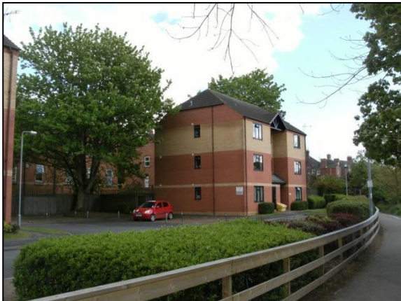
Stonemason's Court, St Catherine's Road.
