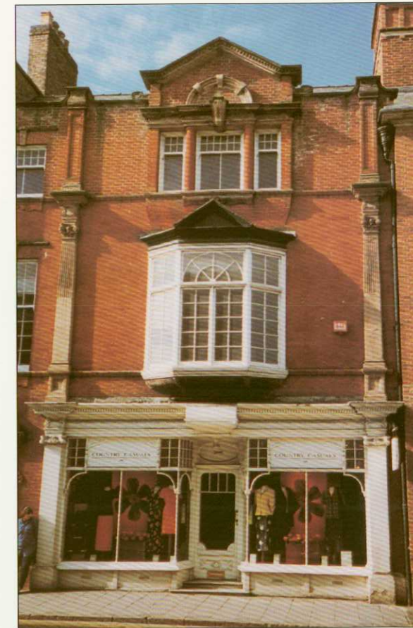
4.6 A full width shop front must appear to adequately support the upper floors
