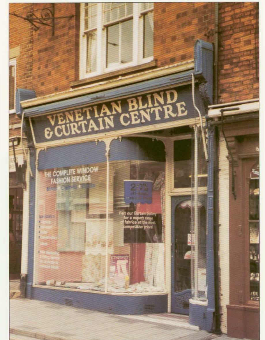
6.1 Traditional blind designed into the cornice
