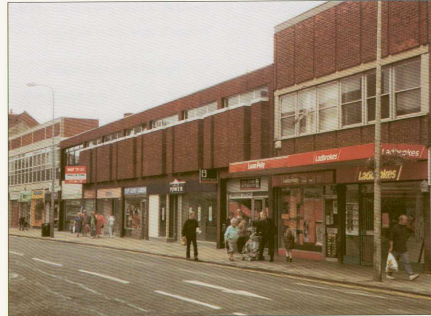
4.4 Characterless redevelopment – a radical approach is needed
