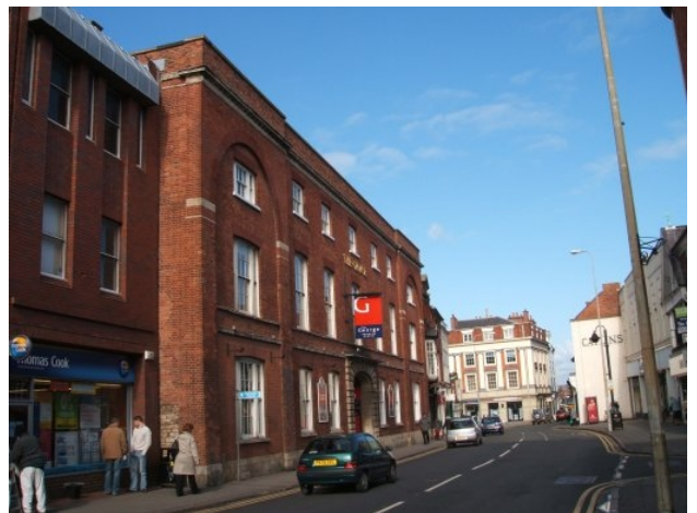
Fig. 10. View northwards along High Street, The George is on the west side of the street with the former National Westminster Bank in the background.
