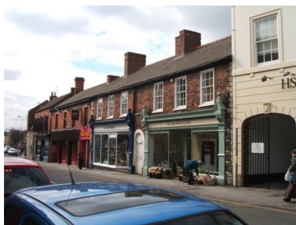
Fig. 12. Examples of traditional shop fronts along Westgate.
