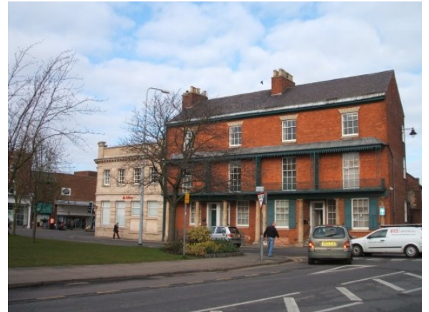
Fig. 19. Numbers 2-4 St Peter's Hill, an attractive example of 19th century Regency style housing
