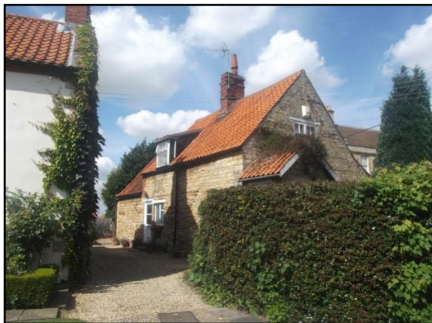
Fig.5 Holly Cottage, Fulbeck (Grade II), typical in its traditional design, one and a half storeys constructed of stone (likely from a local quarry) pantile roof with a steep pitch.
