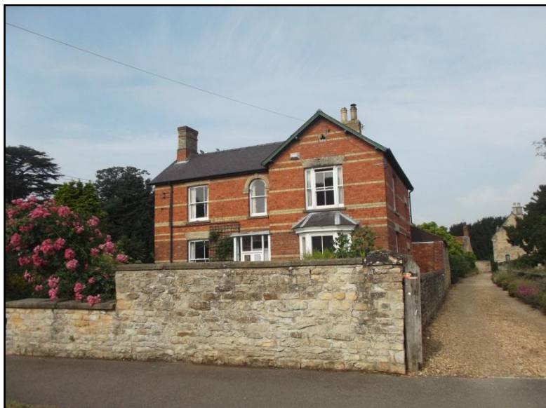
Fig.11 East View, Cliff Road, built in 1885 by Mr Charles Baines, a local joiner, with good retention of original features such as two by two sliding sash windows. The property has a pleasing aspect, adjacent to the open space of St Nicholas Church Yard and looks out onto the rising escarpment to the East, hence 'East View'.
