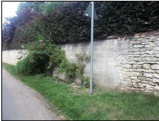
Fig.13 Inappropriate use of block work walling material at Rectory Lane is not in keeping with the character and appearance of the conservation area.
