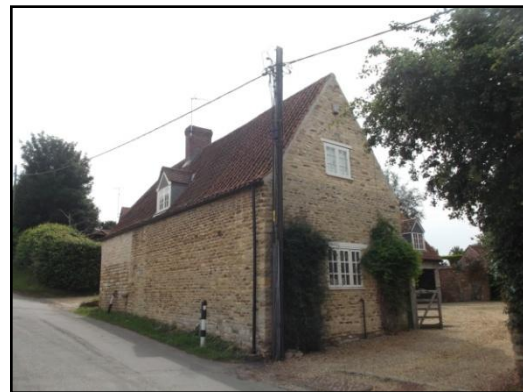
Fig.10 Pickers Mallow, Scotts Hill, a traditional one and a half storey cottage, of rubble construction with attractive plain elevation facing the road. There is a roof dormer which is a common feature on many of the cottages in the village.
