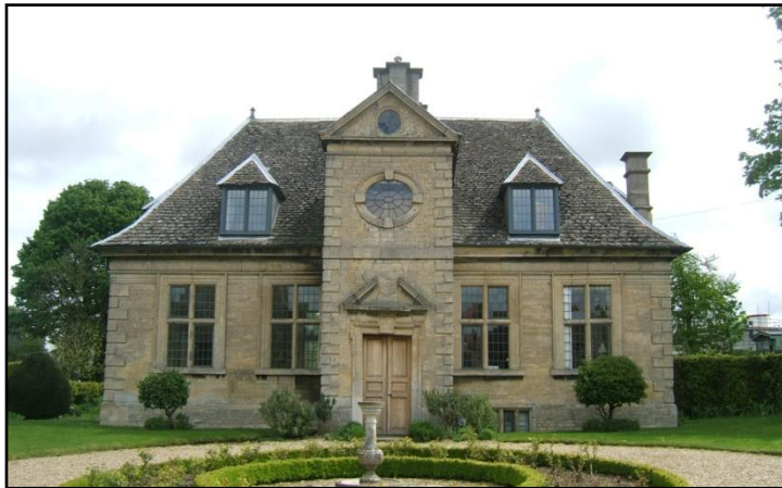
Fig.5 The Grade I listed Willoughby Library and Art Gallery is of exceptional interest and stands prominently within the conservation area at the top of Morley's Lane.
