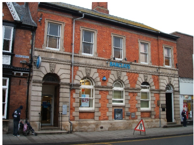
3.1 good traditional shopfronts and unique historic facades should be retained
