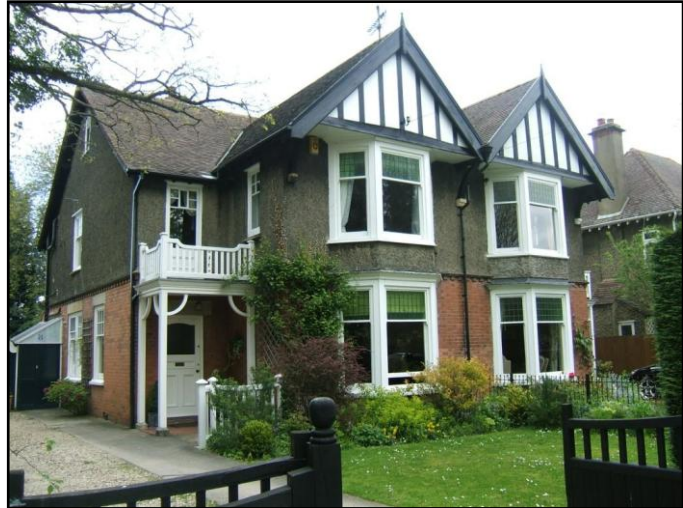
Fig.28 6-8 West Road; Semi detached properties set back within gardens with use of harmonious materials associated with arts and crafts design.
