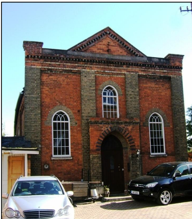
Fig.8 Vestry Hall, located to the rear of North Street with an attractive brick facade is unlisted but makes a positive contribution.
