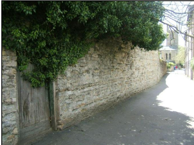
Fig. 16 Boundary walls of random rubble enclose the footway and create visual consistency along Church Walk.
