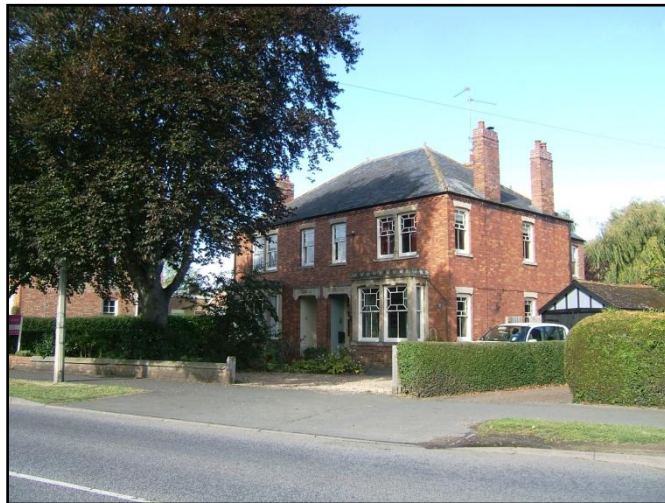
Fig. 29 No.12-14 West Road; an attractive late Edwardian property with refined features.
