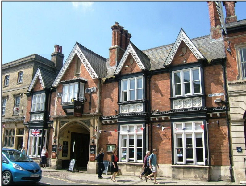
Fig. 2 The Angel Hotel (grade II listed), built in 1880 of a Tudor Style makes a prominent contribution to Market Place.
