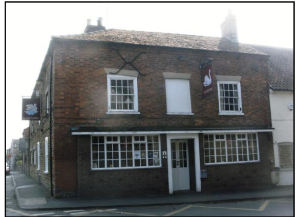
Fig.5 The White Swan Public House: A prominent building at the centre of the conservation area.
