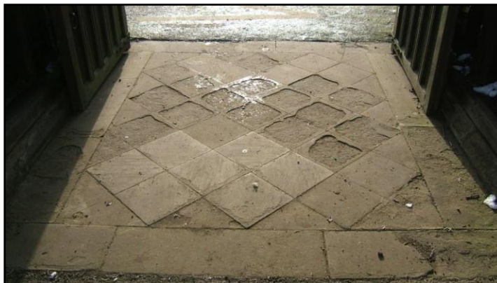
Fig. 14 Weathered diamond shaped flagged floor at Lych Gate of All Saints Church.
