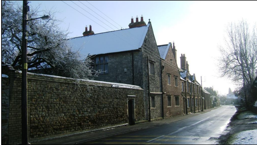
Fig.8 The Grange and adjoining boundary wall Low Road which is aligned close to the footway, deflecting views along the street. The building has two attractive gables, stone mullions and an enclosing boundary wall.
