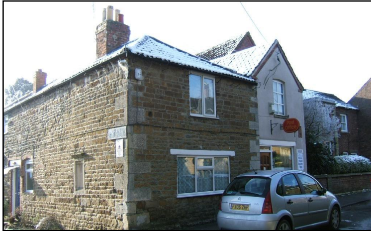
Fig.10 No.1 Chapel Lane and Post Office. The use of ashlar quoins and coursed ironstone is used widely across the conservation area.
