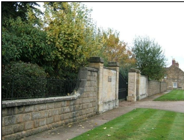
Fig.9 The concrete block walling would benefit from replacement with limestone which is more consistent with the material palette of the conservation area.
