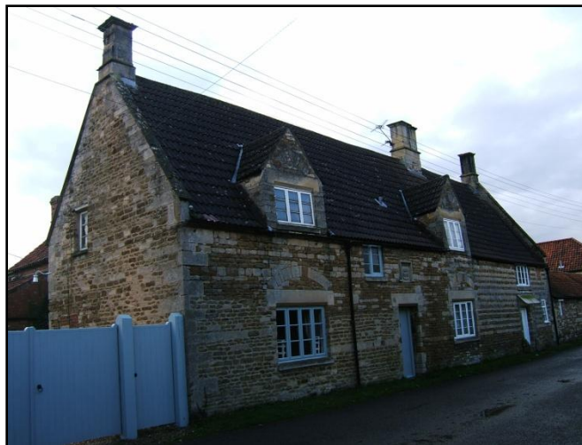
Fig.1 Use of ironstone on buildings in the conservation area adds to the visual palette, such as at The Old Manor House, West Street (Grade II listed)
