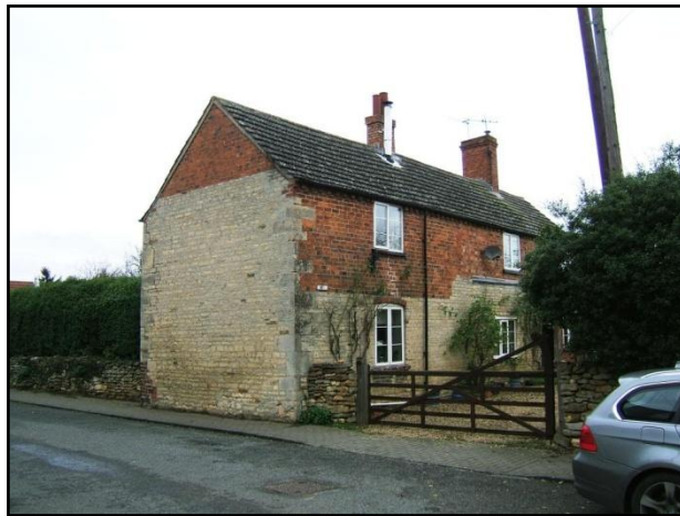
Fig.3 The combination of Random rubble stone and brickwork is a common vernacular approach used across the conservation area.
