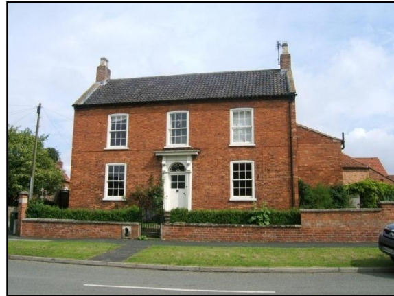
Fig.7 Detached brick properties of the Georgian period, such as The Red House are common within the conservation area.
