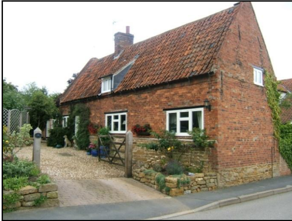
Fig.9 Ilex cottage, a traditional gable end on cottage, with an attractive mix of coursed ironstone and brick contributing towards a warm visual palette.
