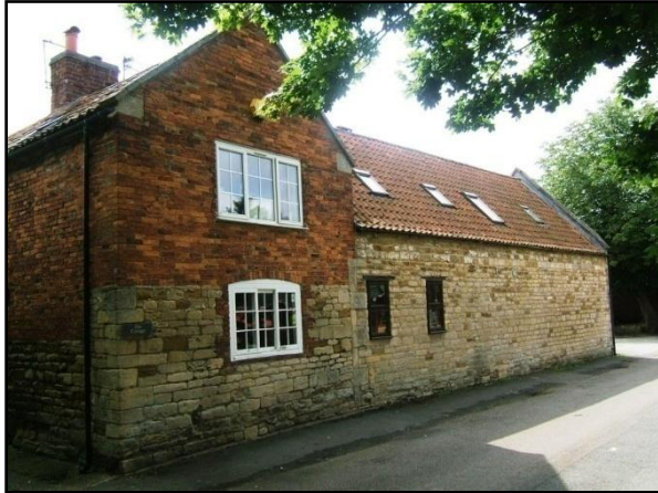
Fig.12 The Old Stables, The Green with an L shaped plan form and an attractive mix of coursed limestone and brick.
