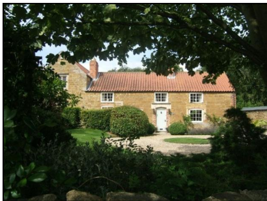
Fig.8 Grade II listed Plum Tree Cottage; built of harmonious material palette of ironstone with red pantile roof
