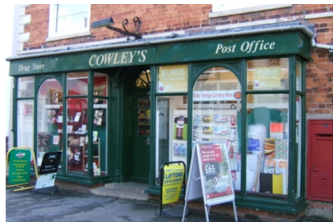
Fig.22 Cowleys Post Office, with attractive shop front is currently being undermined by clutter created by ‘A’ frame boards and unauthorised display of adverts.
