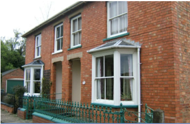
Fig.7 Historic railings at Nos. 9 and 11 Church Street. Dwarf boundary walls and cast iron railings are common across the conservation area.
