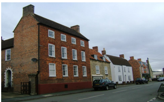
Fig. 1 High Street is the principal routeway into the village with a linear character and buildings directly addressing the highway. No. 46, with three storeys features prominently.
