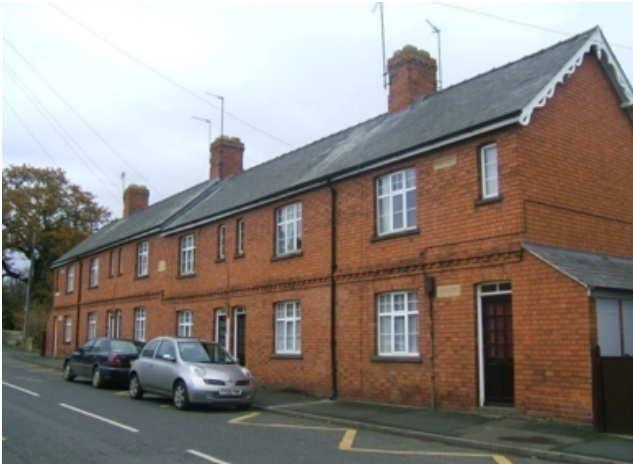
Fig. 13 Nos. 24-34 Low Nests – the terrace has a novel sign inscribed at ground and first floor levels; with 'low nests' at ground floor and 'high nests' at first floor.
