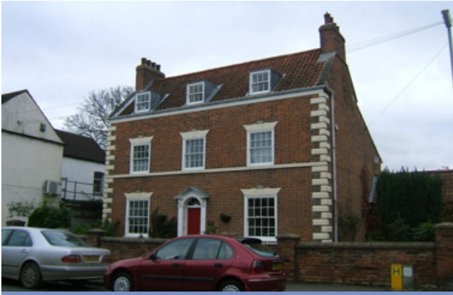
Fig. 6. No. 70 High Street, with 'moustache' lintels, that are typical of the conservation area and are common in other fen margin villages.
