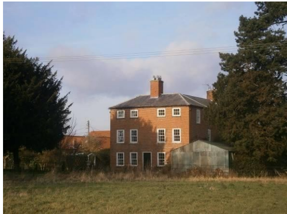
Photo of Brandon Hall, the only three storey building in Brandon indicating its historic importance and prominence within the village.
