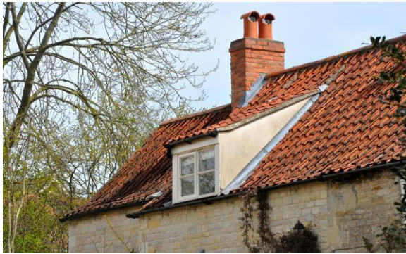
Red pantile roof and Cat Sled Dormer window
