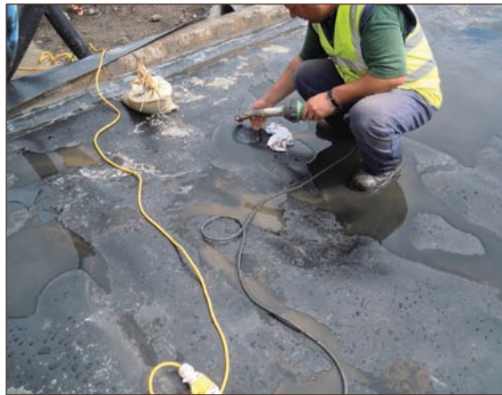
Figure A4.40 CO 2 injection integrity testing (courtesy Landline Ltd)
