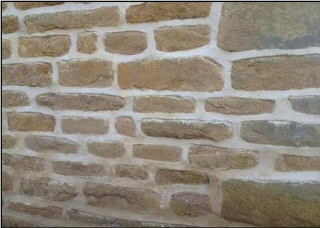
*Inappropriate weather struck and ribbon pointing can cause both visual and structural damage to both brick and stone masonry*
