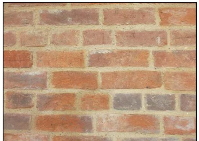
*Example of good repointing work, with flush joints using a lime rich mortar with graded sand.*
