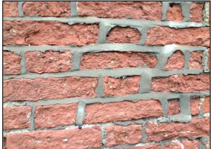
*Hard cement pointing significantly detracts from the appearance of a historic building and traps moisture within the walling causing damp*
